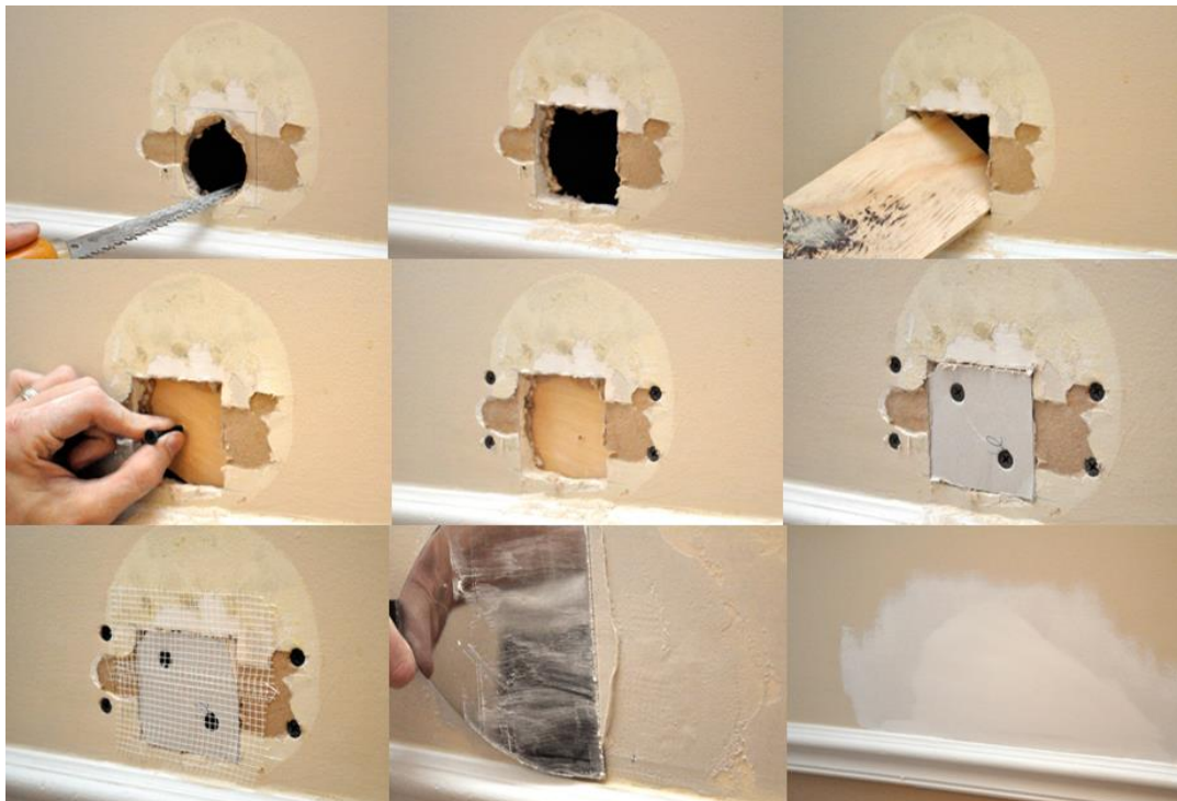
Figure 1: Sheetrock hole repair. Ethan. 1 June 2018. One Project Closer, How to Repair a Medium-Size Hole in Drywall, https://www.oneprojectcloser.com/how-to-repair-medium-size-hole-in-drywall/ .
